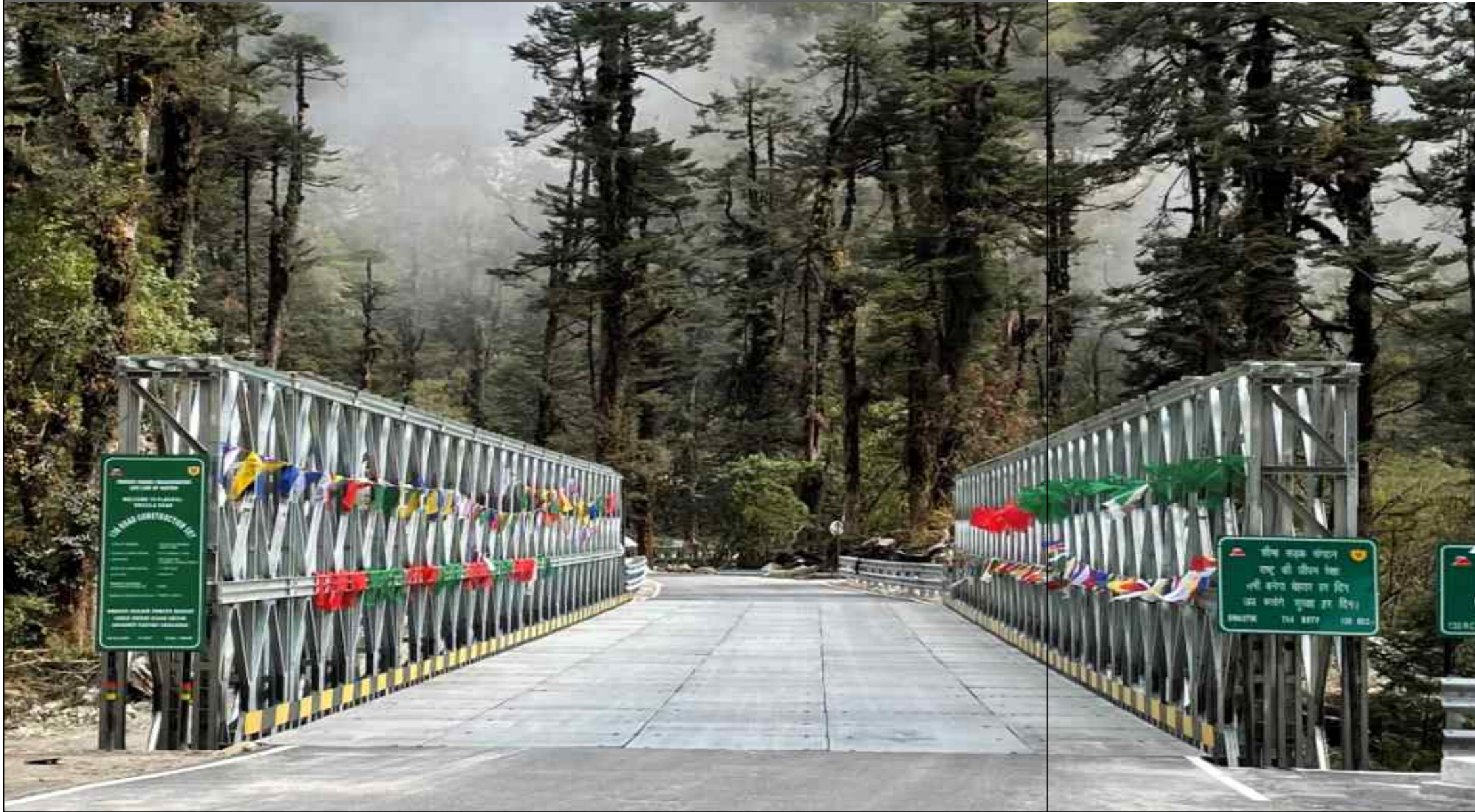
CL-70 Double Lane Modular Bridges on Flag Hill-Dokala Road
