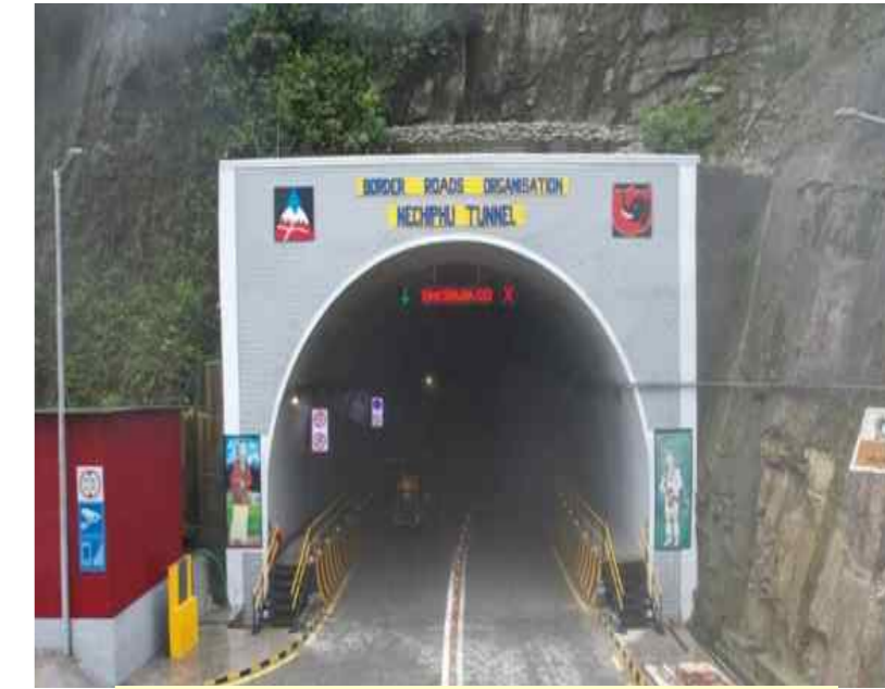
500 m long Nechiphu Tunnel on Balipara Charduar Tawang Road
