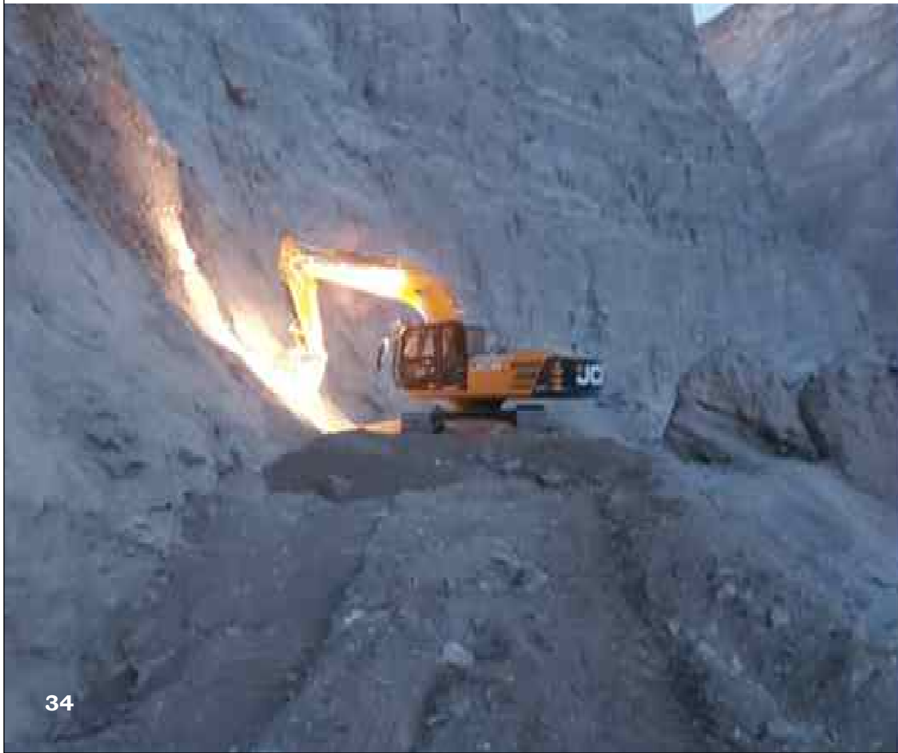
Fmn Cutting in Progress between Chilling & Niraq and Kilima & Niraq
