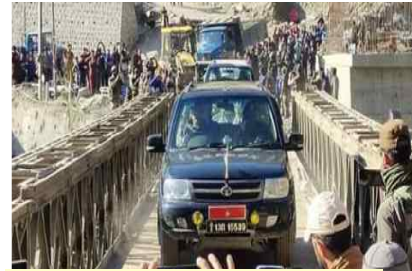
Bridge of Assistance (Kela Bridge, Jammu-Srinagar Highway)
