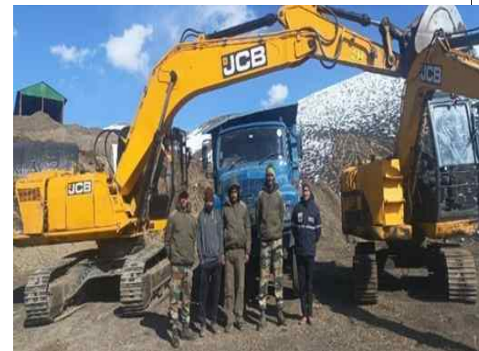
Connectivity achieved on Sumna-Lapthal Road
