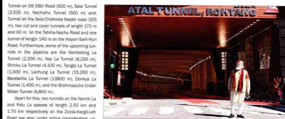
zone of each length (587.5 m) had never been encountered in a single stretch of any highway tunnelling project in the world before, and took almost four years to overcome. From change 1,387 onwards, the quality of rock started deteriorating, and at change 1,950, the condition of the face became devoid of rock. Muck, along with water, started flowing from the face inside the tunnel due to the weathering caused by Seri Naha's discharge from its natural course to the South Part of Atal Tunnel.
